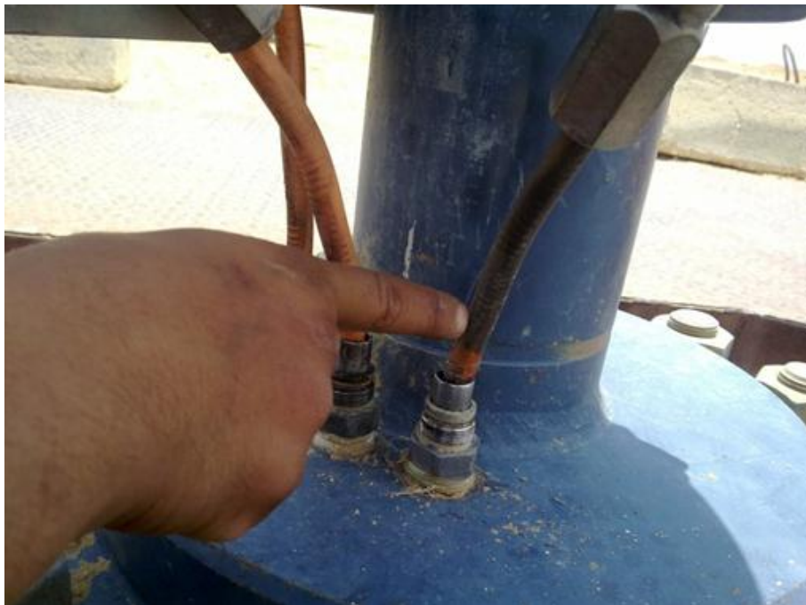
Figure 4.10 Cable electrical short
