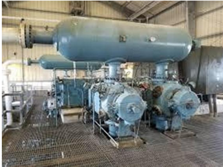
Figure 2-36 Reciprocating compressors
