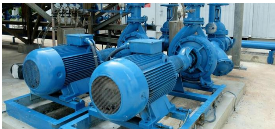
Figure 2-42 Centrifugal Pump
