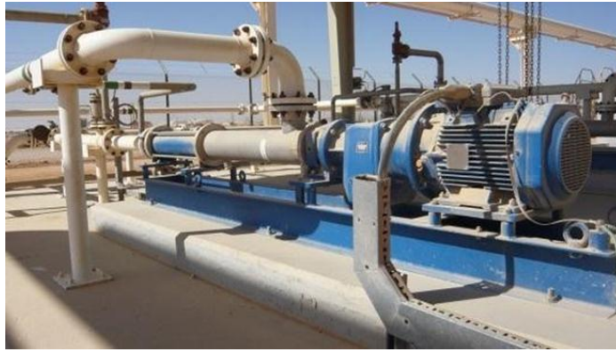
Figure 2-44 Oil Transfer Pump
