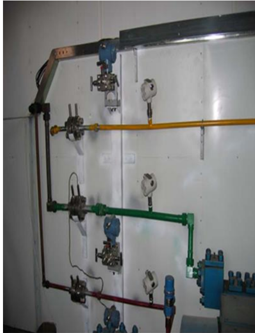
Figure 4-4 Flow lines for feed oil, water and air
