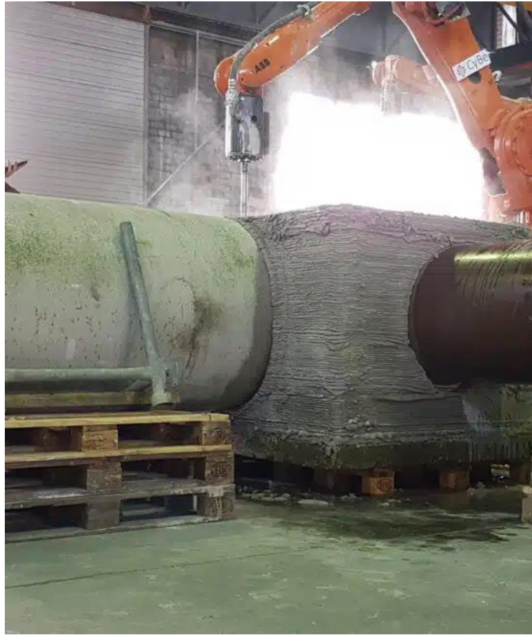
Figure 7-14 3d printed manholes[62]
