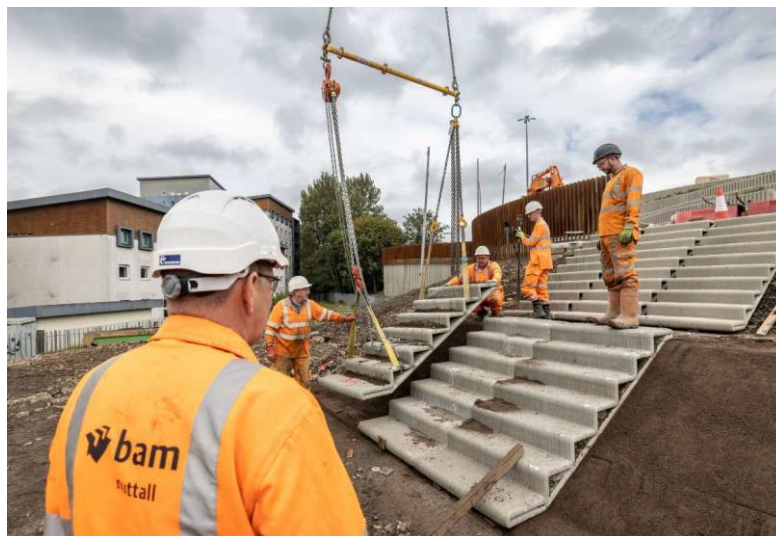
Figure 7-19 Concrete Stairs From 3d Printer[67].
