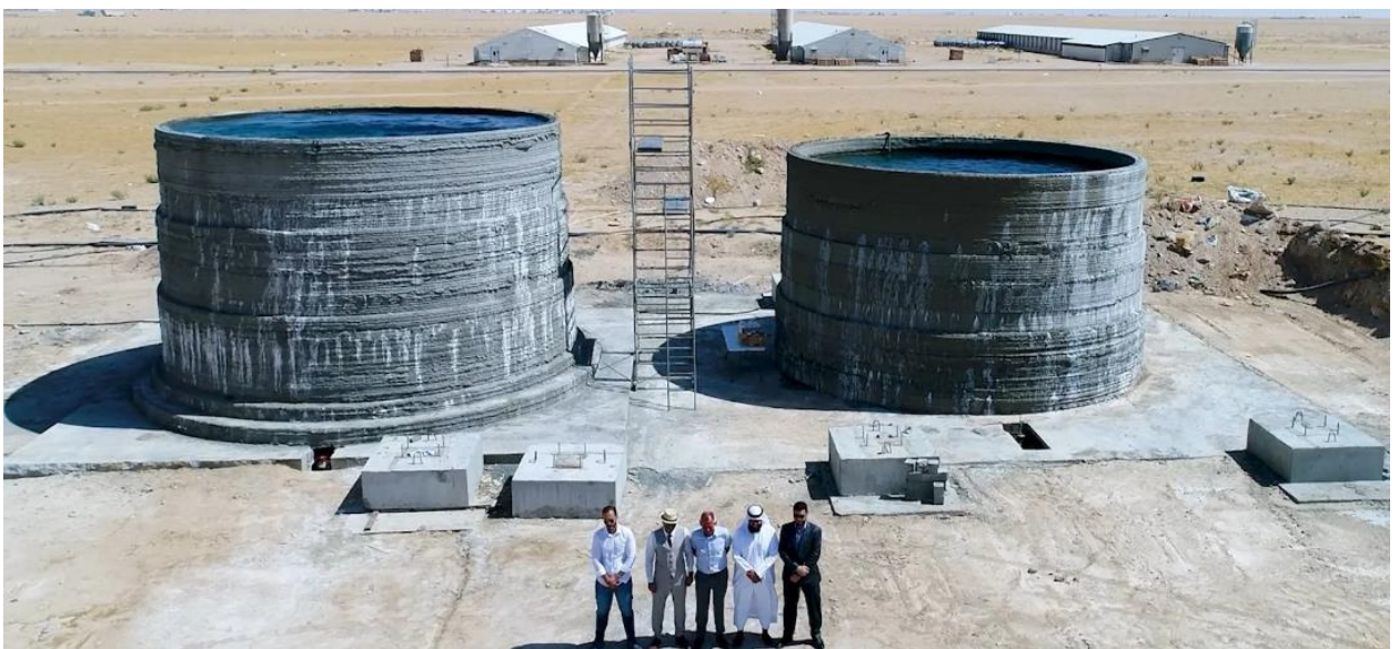
Figure 7-15 3D-Printed Water Tanks for Kuwait United Poultry Company[63].
