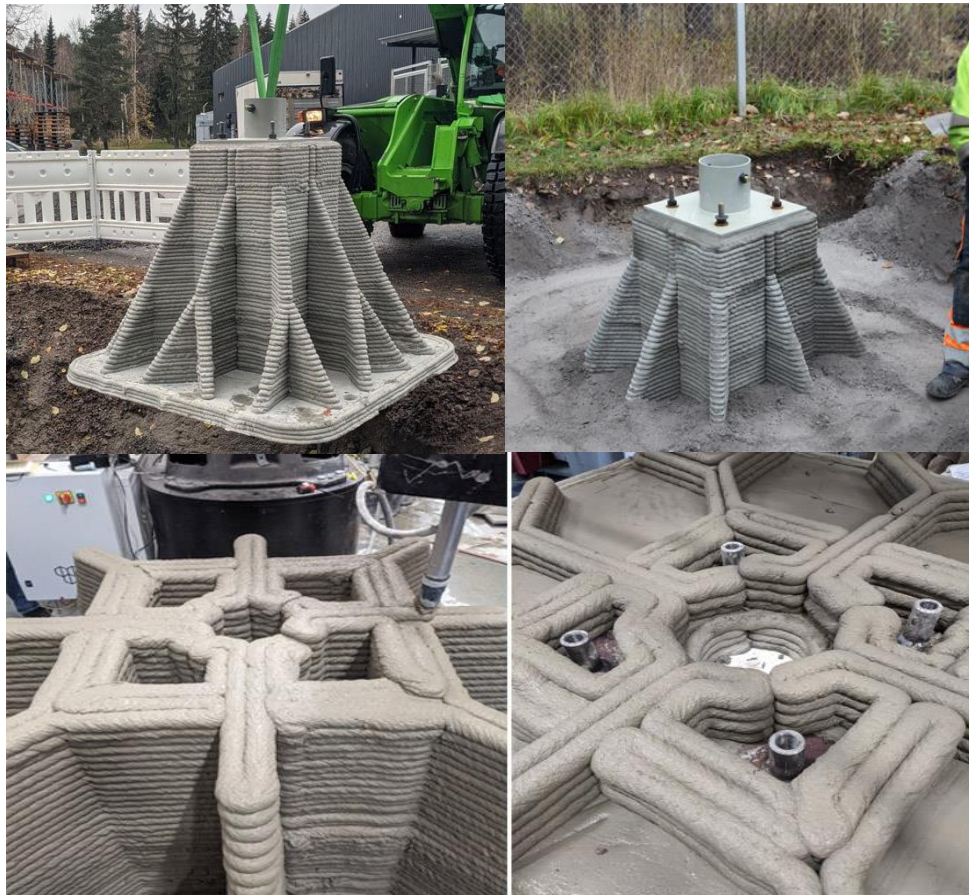
Figure 7-18 3D-Printed Energy Infrastructure With Lower Material Consumption[66]
