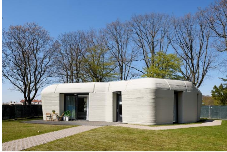
Figure 1-5 The house was built using concrete 3D printing technology under the Milestone project in the Netherlands [2].
