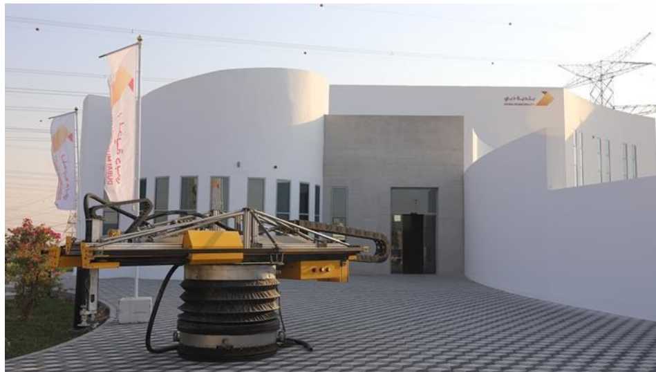
Figure 1-1 The building was constructed using a concrete 3D printing robot in Dubai developed by the company Apis Cor [1].
