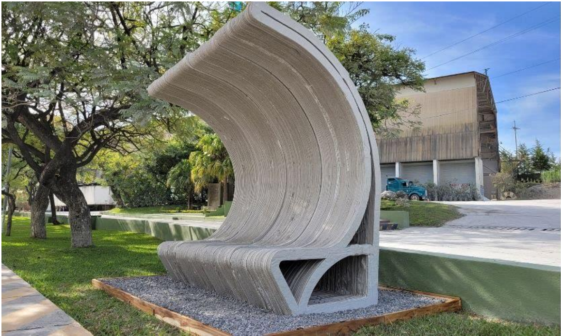
Figure 7-24 3d printed stop chairs
