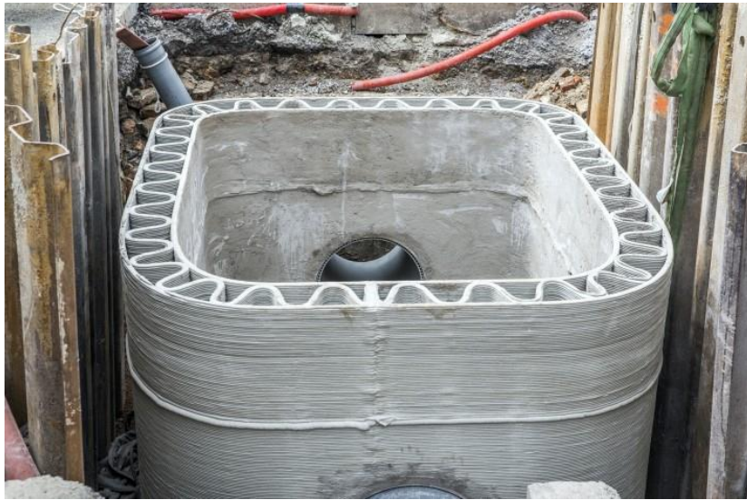
Figure 7-13 3d print drainage[61].
