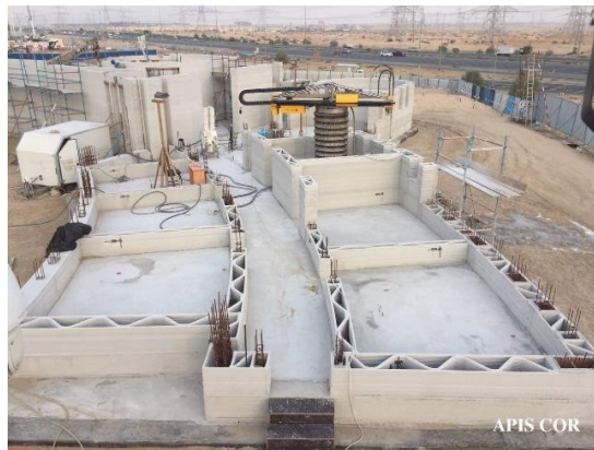
Figure 1-2 The wall of the building is being constructed using the 3D printing method [1].
