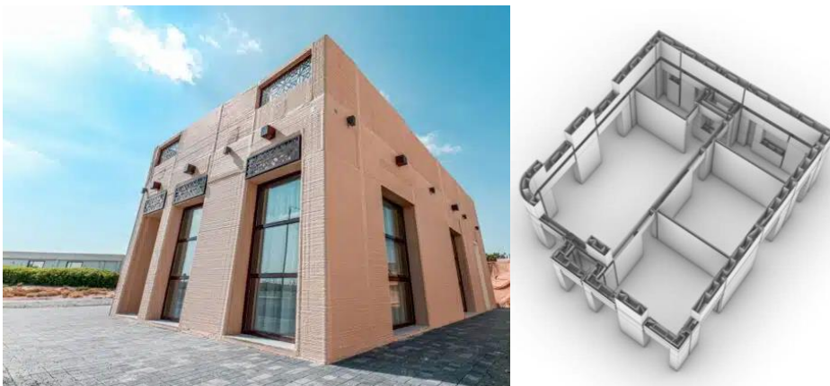
Figure 7-2 3d Concrete Printed Villa in UAE[54].
