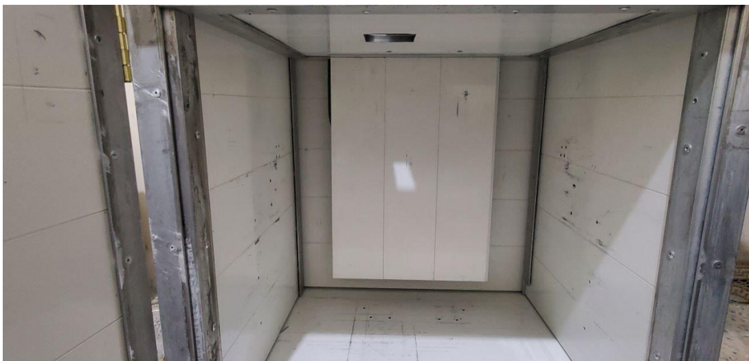
Figure 4.16 Use of private sector aluminum to build an insulating wall between the hot file and the printing chambers and the store to avoid direct heat reaching the printing bed.
