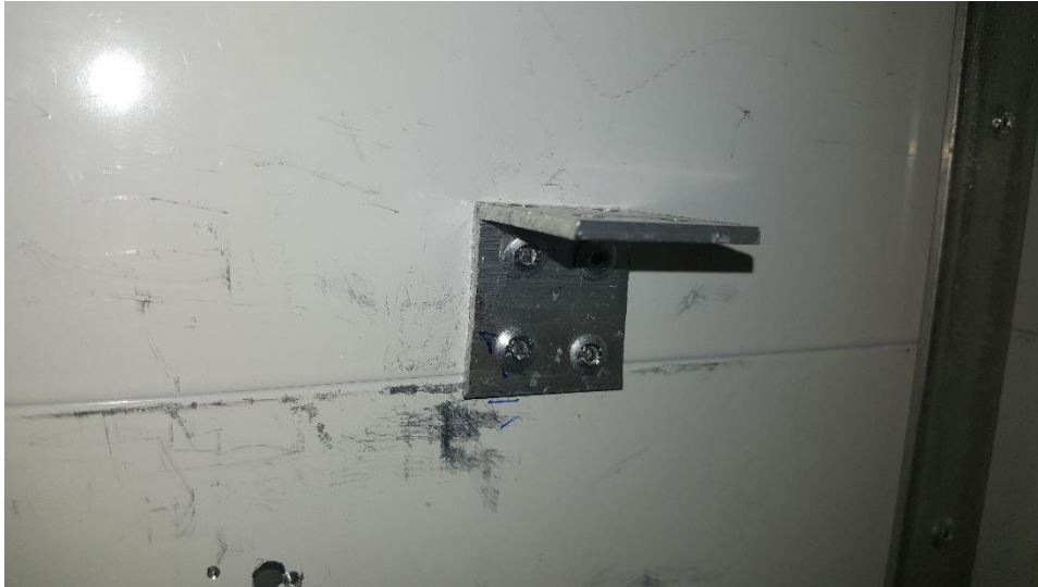
Figure 4.18 example of using aluminum at a 90 degree angle in a place to raise the printing rooms and the warehouse, after it was cut with a saw and its edges were smoothed
