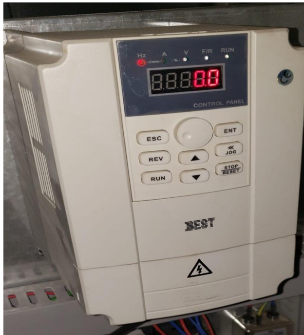
Figure 3.7: Inverter 3.5kw
