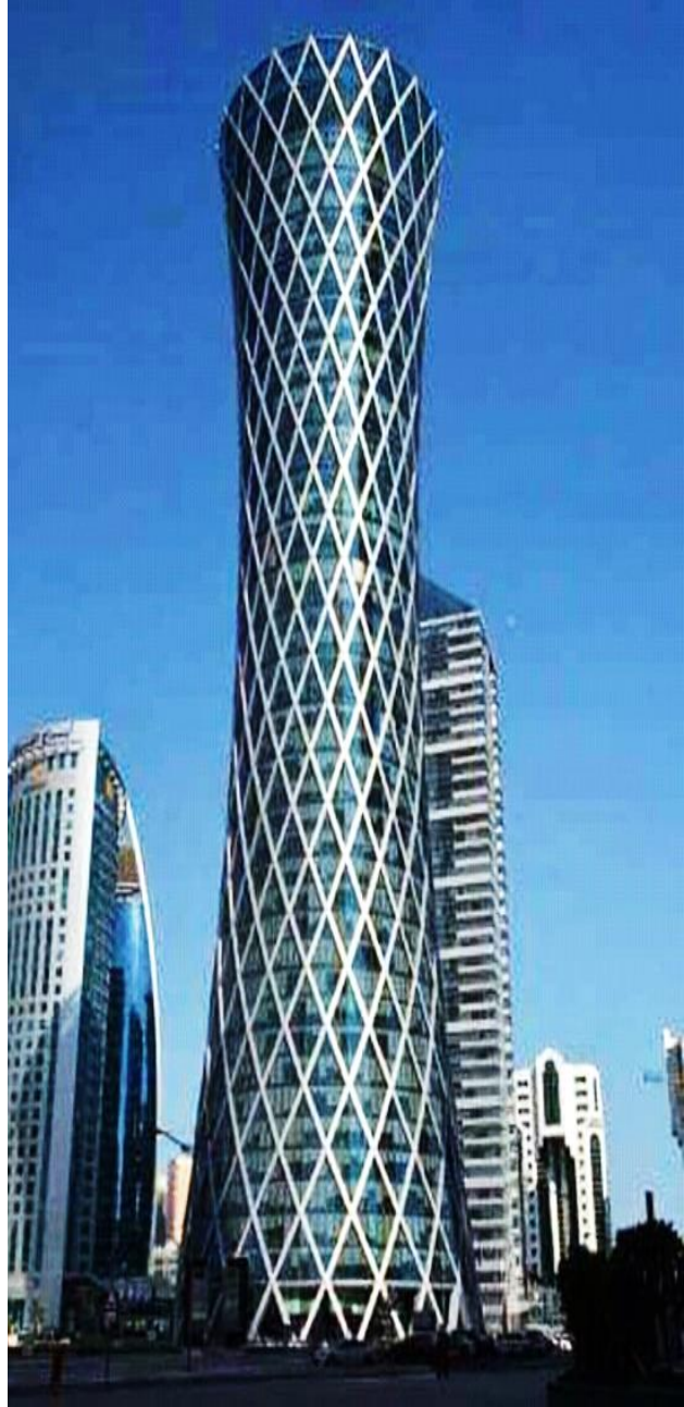
Exterior diagonal braces in a tall steel building.
