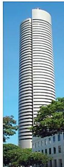
Reinforced concrete mega core (circular cross-section with external diameter of 25m and varying wall thickness of 1.65 to 1m from bottom to top)
