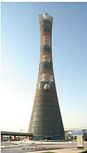
Reinforced concrete mega core (circular cross-section with varying external diameter and wall thickness of 18 to 13m and 2 to 1m respectively from bottom to top)
