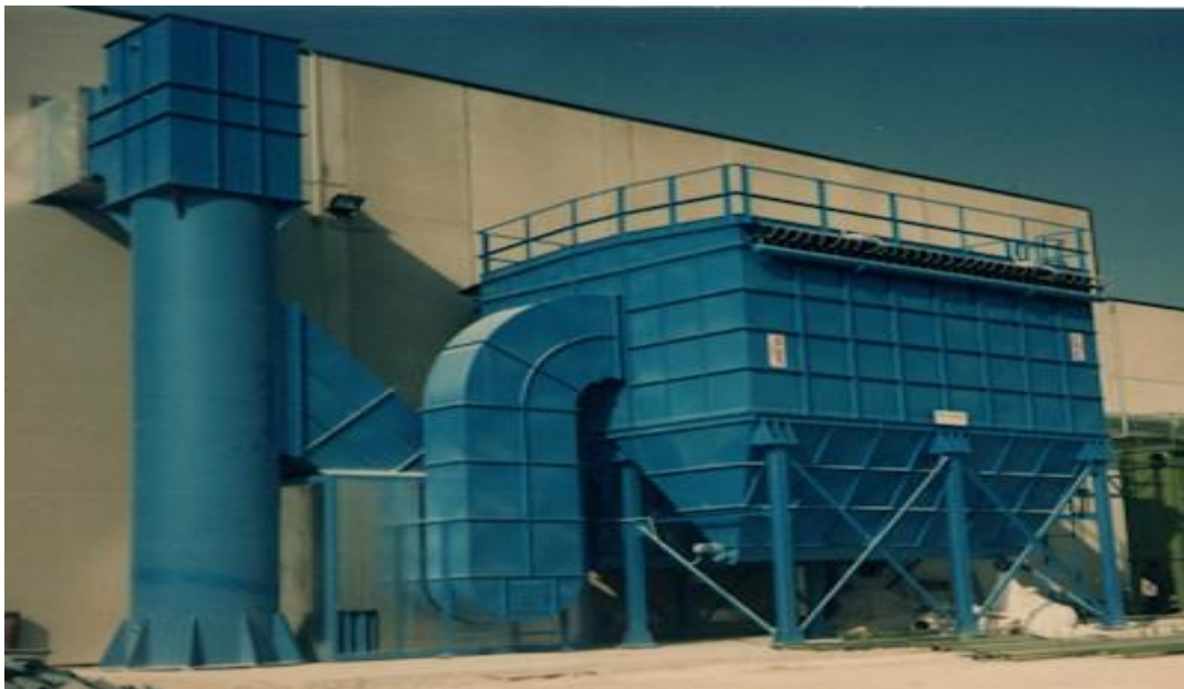
Figure 5.8 Filter Baghouse
