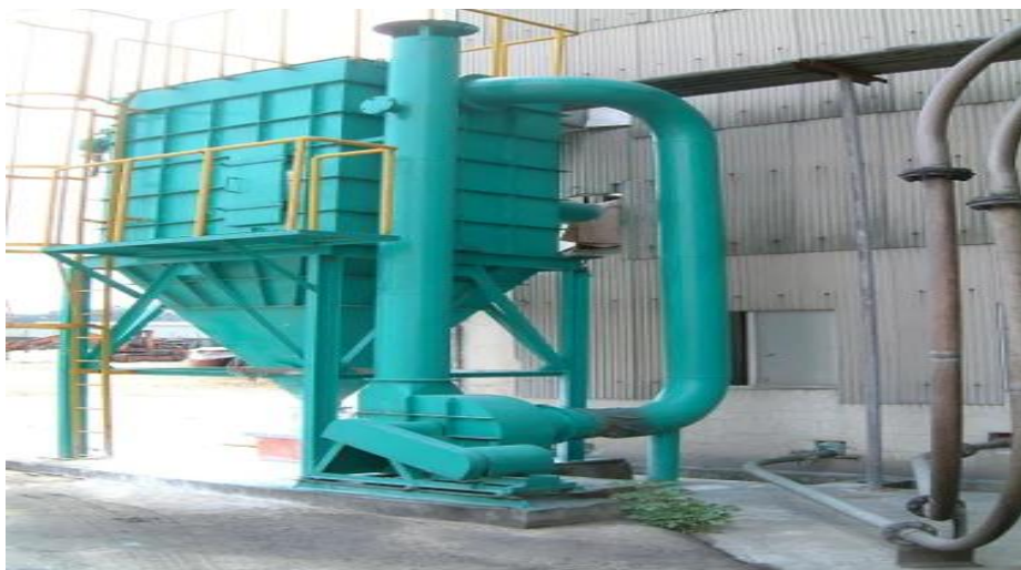
Figure 4.4 Filter Baghouse
